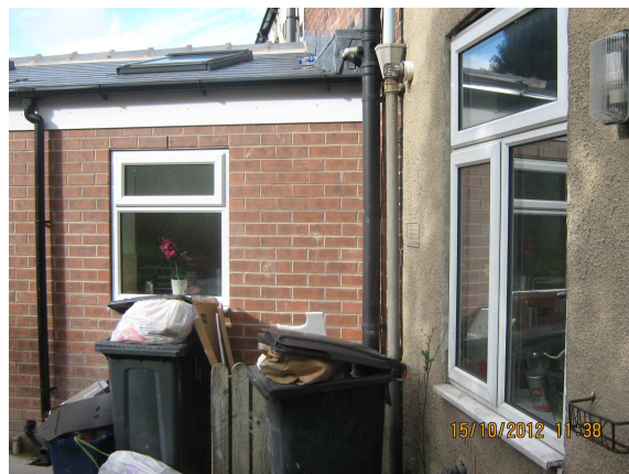
Photograph 3 Clear glazed window overlooking the rear of No 27
